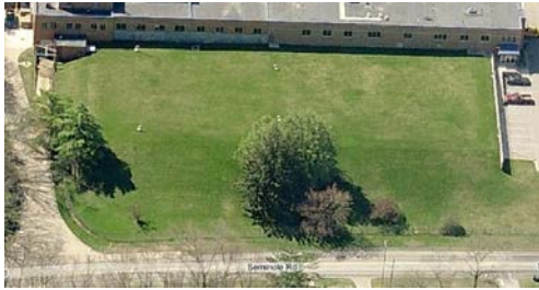
WTP East and West Reservoirs
