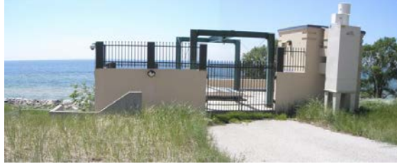
Low Service Station
