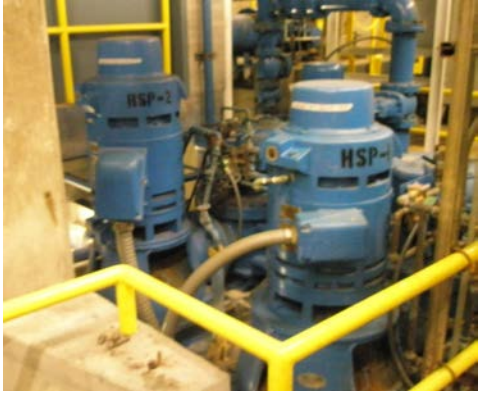
WTP Old HSP No. 1 & No. 2
