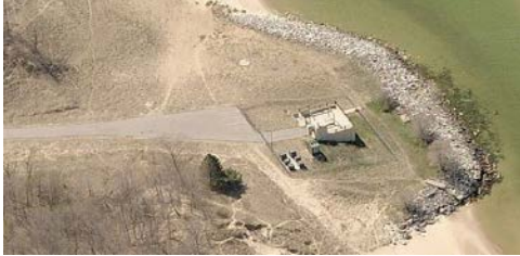
Low Service Station Aerial Photo
